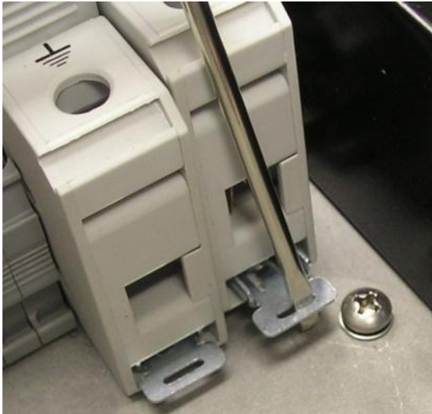
Figure 5-6 – Remove Surge Suppressor Assembly.
