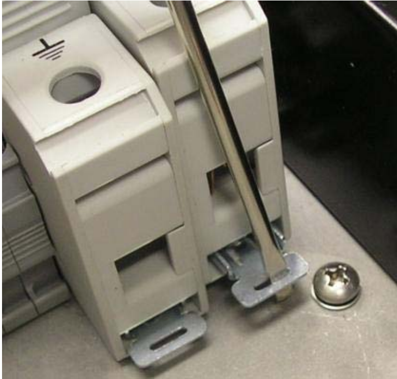
Figure 5-6 – Remove Surge Suppressor Assembly.
