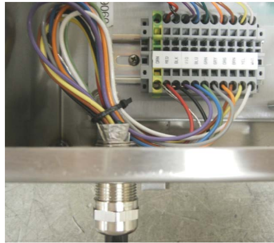
Figure 2-2 – FH Cable Install (PC)
