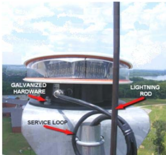
Figure 2-5 – FH Mounting
