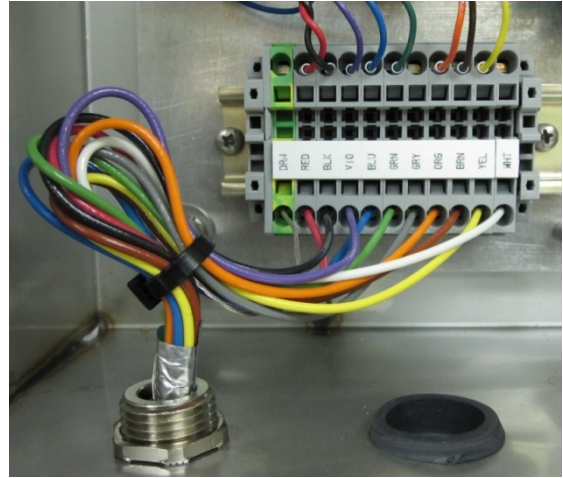
Figure 2-2 – FH Cable Install (PC)
