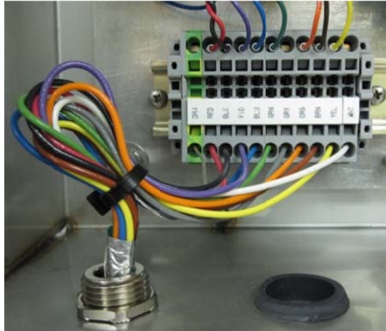
Figure 2-2 – FH Cable Install (PC)
