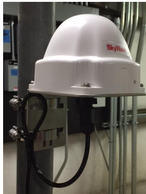
Figure 4-7 – Pole Mount Installation
